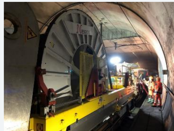
Zimmerberg tunnel CFF
