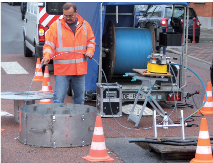
Blowing of microcable in mid-span technic, using the Figaro.
